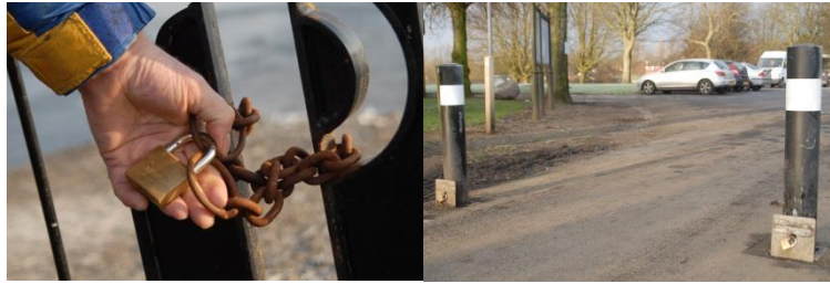
Gate/fence at Kelvingrove Park/River Kelvin repaired
