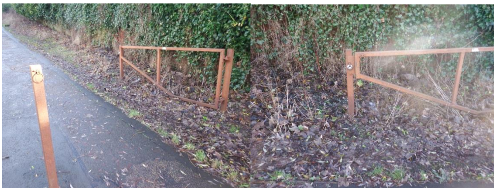
Boom gate at Belvidere east repaired
