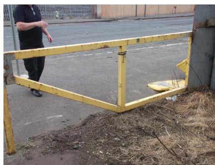
Boom gate at Belvidere west repaired
