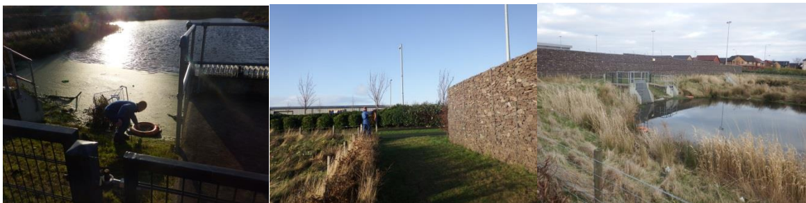
Extra emergency and maintenance access gates on riverbank fencing throughout Glasgow Green
