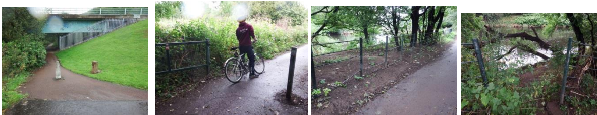
Bollards prevent access Boom gate open Gap in fencing Gate missing
