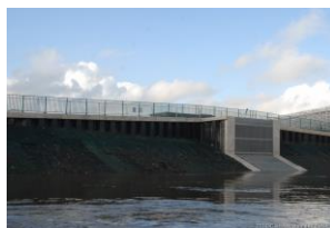
Wall covered at high tide
