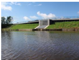
Outflow showing concrete wall.
