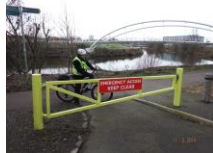
Boom gates give emergency access. Also prevent fly tipping and vehicles being driven into the river.
