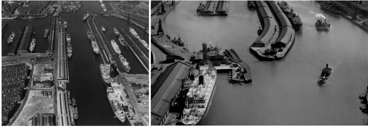
The mainstream of the river Clyde has been narrowed. It used to be mostly wooden jetties out into the river above a sloping bank that allowed overspill, a wider river, at times of high tide.
