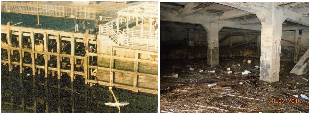
It is now mostly piled quay wall. The upper harbour of the Clyde has not been dredged for years and is now up to 6m shallower in places. Large mud flats show at low tide where the iron ore ships used to berth.
