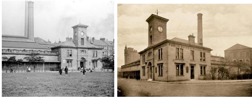
Greenhead Public Baths and Wash-house in William Street (later Templeton Street) in the early 20th century.
