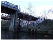
The deck of the old bridge was removed and the second phase started
