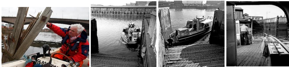
Ferries bouncing off dolphins rather than hitting and damaging the quay walls.
