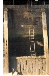
Fenders protecting quay wall. Fenders protecting ladder.
