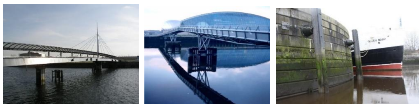
Pier protection Bells Bridge. Millenium Bridge. Wooden protection fenders at dock mouth.
