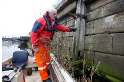
Fenders protecting quay wall. Fenders protecting ladder.
