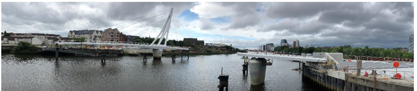
Fenders/Dolphins, on our newest bridge.
